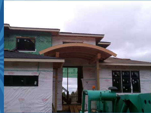
Radius front laminate beams were custom made for front entry
