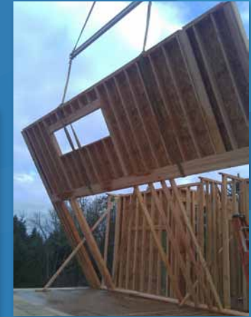
Cranes were used during construction to expedite the framing stage
